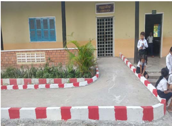
Photo: Ramp and toilet renovation and Phnom Touch
