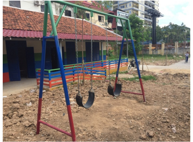
Photo: School renovation 1 building, 5 rooms, 10 classrooms, 1 tiled brick playground with 1 slide, 1 balance, 1 swing, 2 toilets, 2 ramps, 9 trees, 1 rubbish bank, in Toul Kork primary school ,Phnom Penh.
