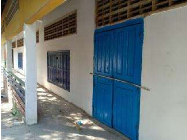
Photo: School renovation (interior painting)
